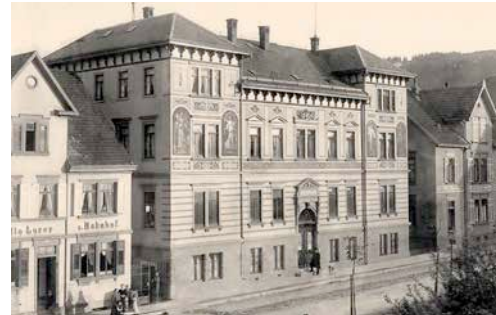
Factory building, Theodor Groz & Söhne in Albstadt, 1884
